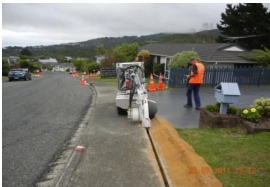
Duct and cable installation
